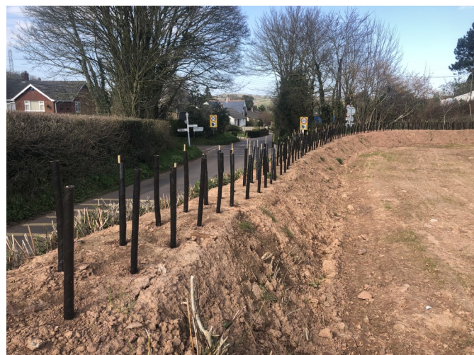
A hedge on hedge bank constructed as part of a previous auction
